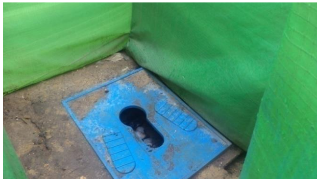
Plate 3: Shallow Latrines Used by Displaced Community in Riziwani Street Provision of Basic services (Water and Health) in the Displaced Community
